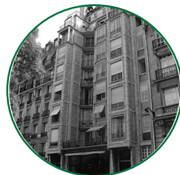
FIRST APARTMENT BUILT First apartment building using steel-reinforced concrete. Built in Paris, France.
