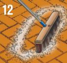
Regular sand option: Sweep coarse sand into all spaces between the finished pavers, repeating the process until all joints between the pavers are filled. Repeat this process with more dry sand in a few days.
