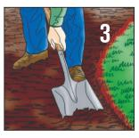
Using your grid work of stakes and guide strings, excavate material below the string lines to the depth needed. To determine depth, refer to the Excavation Depth Guide. Note: Before any digging, call 811 for the location and depth of underground utilities...
