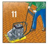
Sweep off the surface completely and use the plate compactor to tamp the pavers to a uniform level. Run the compactor in a parallel direction across the pavers. overlanging on each pass. Make a second series of passes in a perpendicular direction. Important: for large profile pavers or a raised surface paver, set compactor to half speed and use a protective pad to prevent marking and scuffing pavers..
